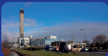
A CHP generator
