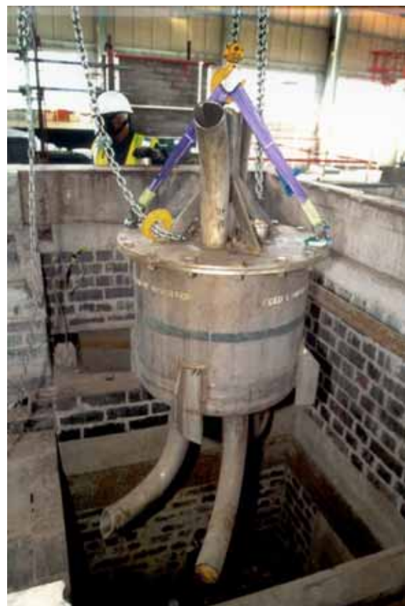
Figure 6: Decommissioning activities at Sellafield (source: BNFL)
