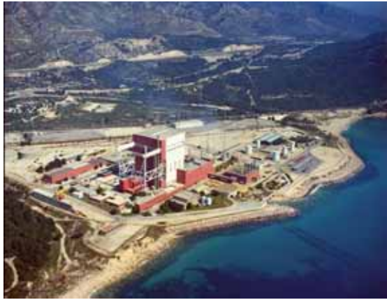
1. General view during operation
